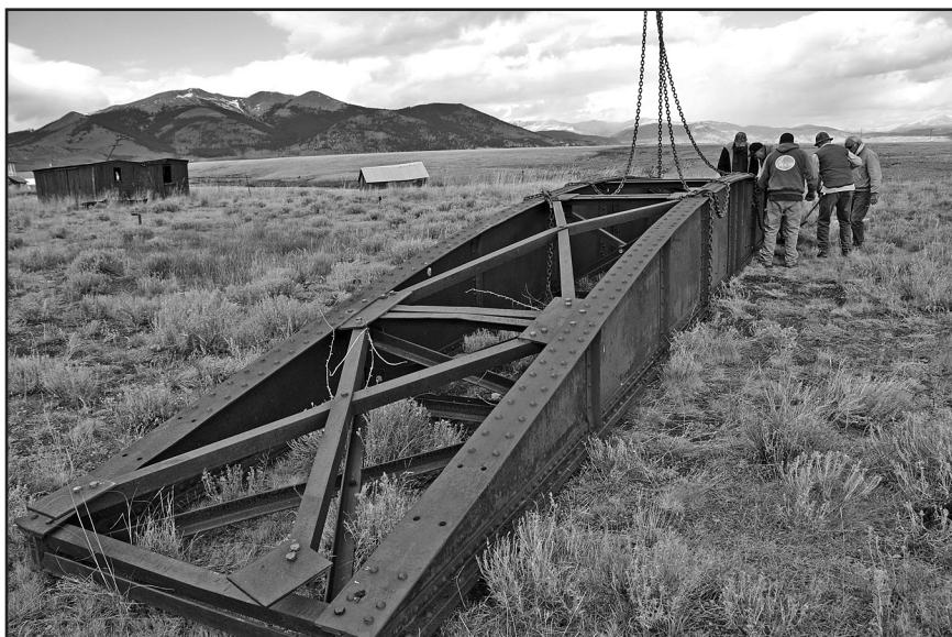
During demolition of a Denver building, Bill Kazel discovered the original Como roundhouse turntable and had it returned to Como. – Photo © 2014 Ann Lukacs.
