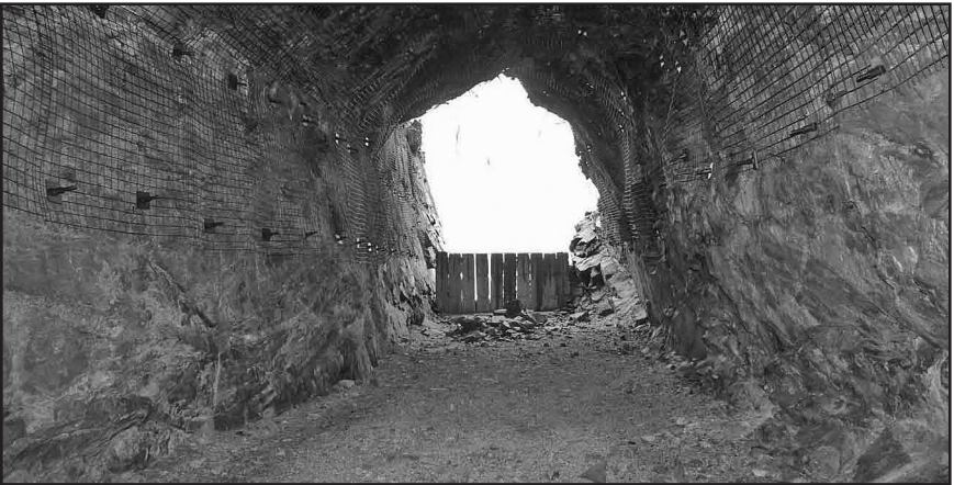
Inside Needle's Eye Tunnel in 2012. – Photo Courtesy of Rollins Pass Restoration Association and Deere & Ault Consultants, Inc.
