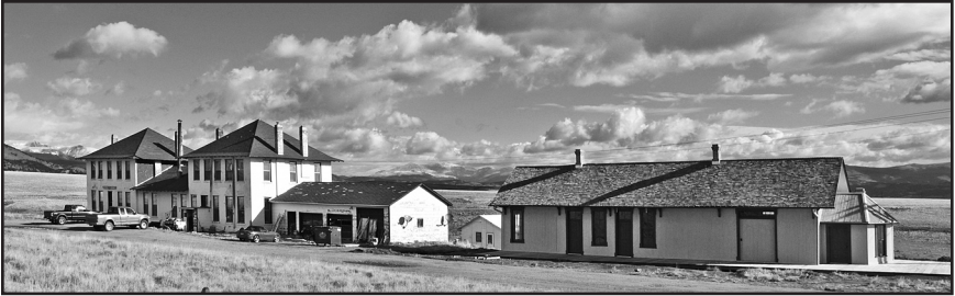
The Como eating house and the depot where restoration is well underway. – Photo © 2014 Ann Lukacs.
