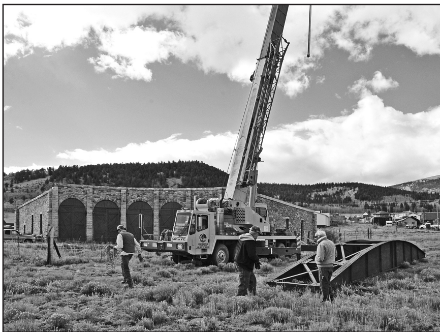
Preparing to place the Como turntable in position. – Photo © 2014 Ann Lukacs.
